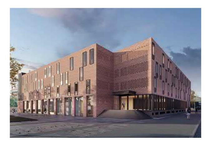
The project involves the extension of an existing building and the construction of a new student residence. The new building will be composed as a single C-shaped body and will consist of two underground levels and four above-ground floors, with a total area of approximately 13,000 square metres and 165 rooms (245 beds).
