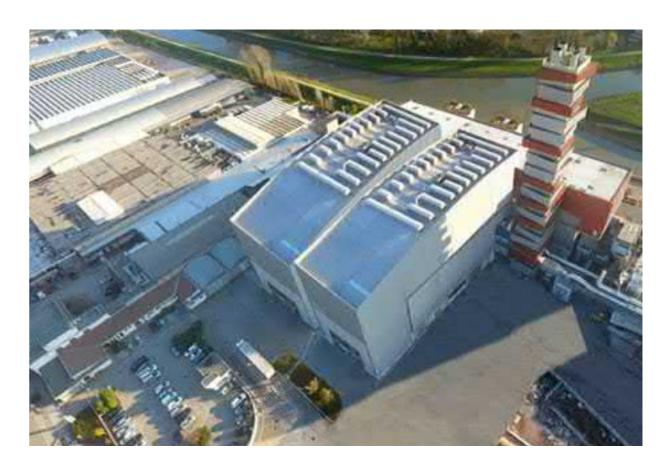
The project involves the construction of the new line 4 of the waste-to-energy plant (WTE) in Padua, with the same capacity as the existing line 3, and all necessary ancillary and related works. Specifically, the contract covers the executive-construction design and execution of civil works and BOP (Balance of Plant).
