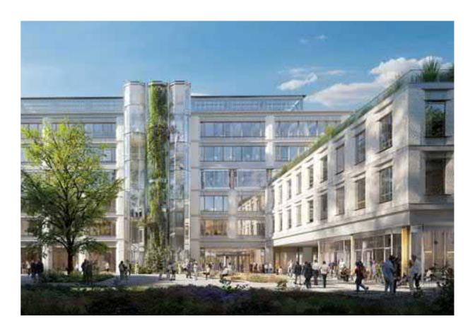
The project "Lorenzini 8" involves the construction of a new office building south of Porta Romana railway yard. This includes two basement floors and two above-ground buildings, totalling 32,500 square metres. The L8A building will have six above-ground floors and L8B will have 5, with reinforced concrete structures and prefabricated panel façades. The project aims to achieve LEED, WELL and WiredScore certifications, using C2C-certified materials.
